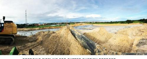
DREDGING PIPELINE FOR CUTTER SUCTION DREDGER
